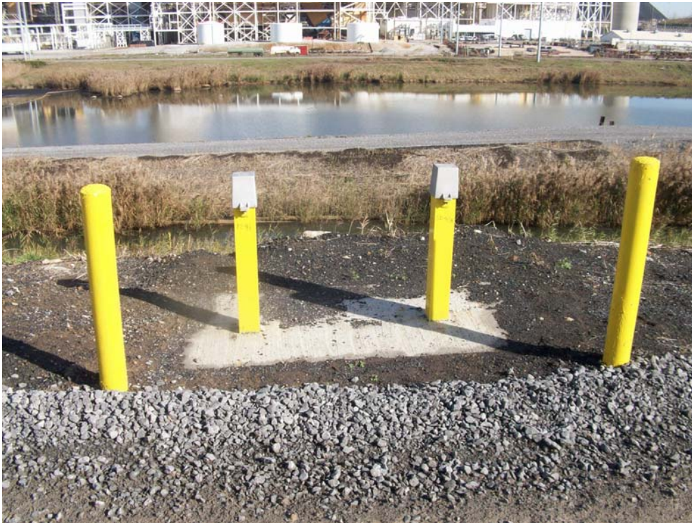
Figure 5. Typical Instrumentation (Slope Inclinometers, Piezometers) Installation
