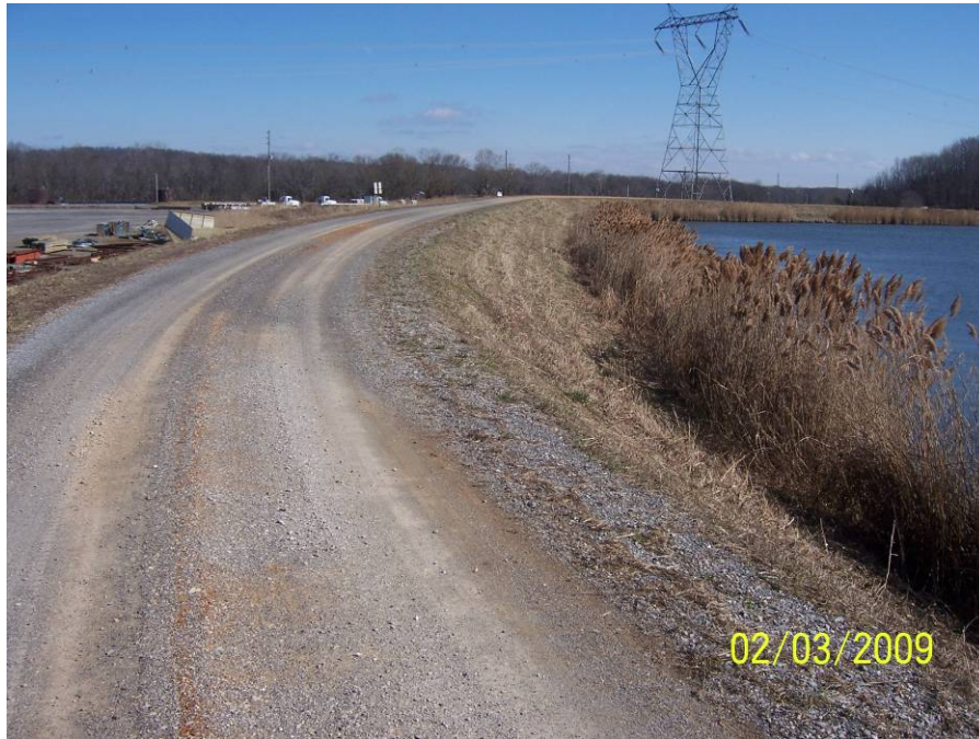
Drawing Mark AP-1-1 Crest and inside slopes of the perimeter dikes around the Ash Pond.
