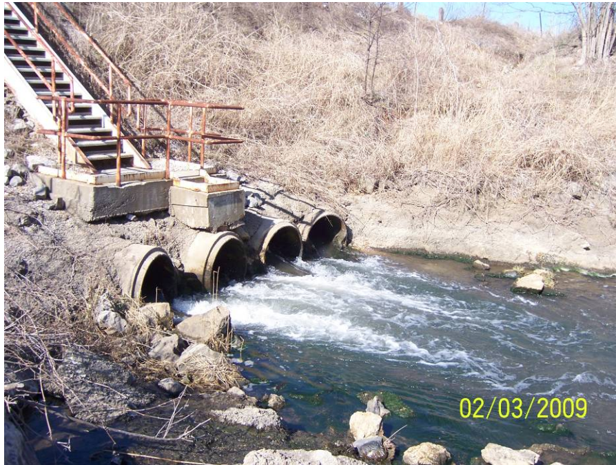
Drawing Mark AP-1-5 Spillway discharge and channel.
